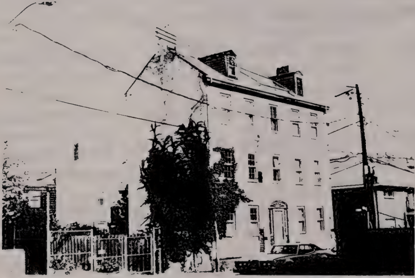
Union st - main facade
